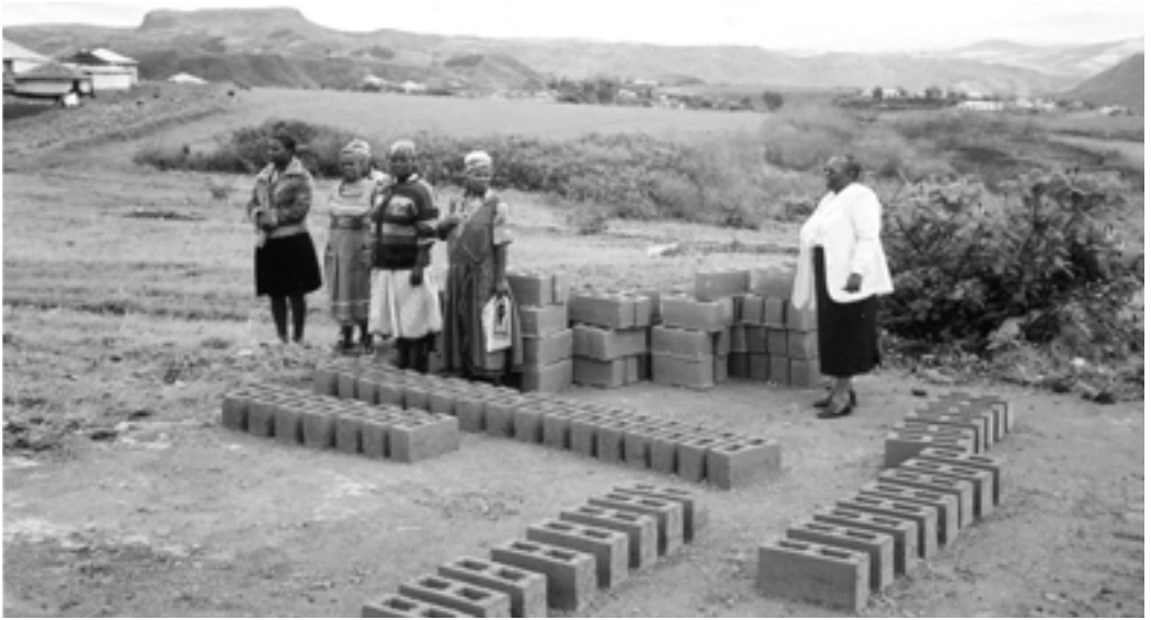
Above: DSE students making bricks
